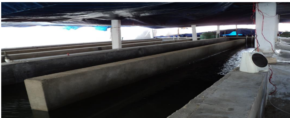
Figure 3.16. Seawater Storage and Filtration Tank (NIMA, 2020)
